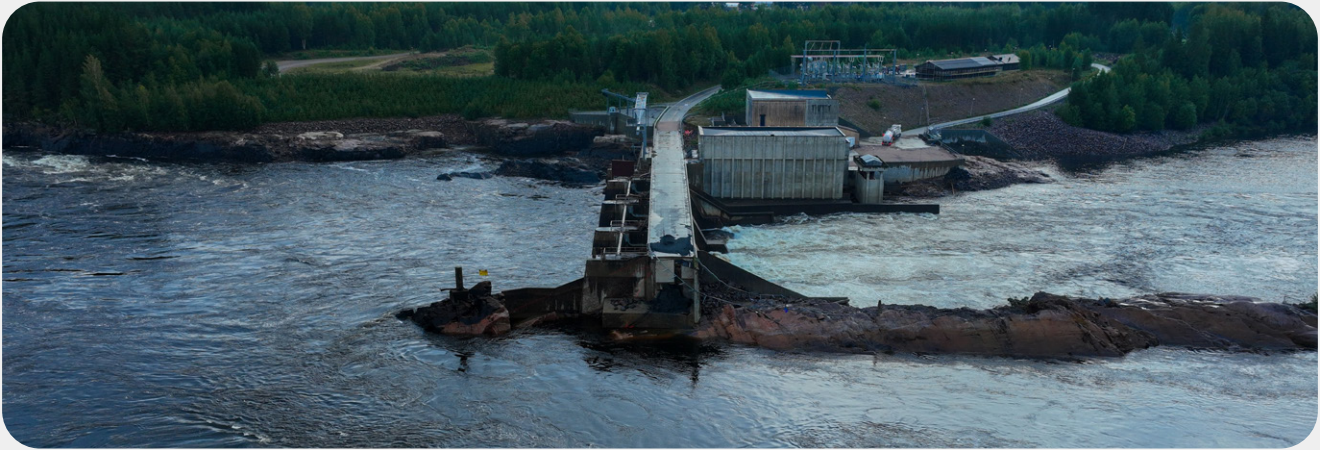
The dam at Braskereidfoss following Storm Hans. Photo: Shutterstock
